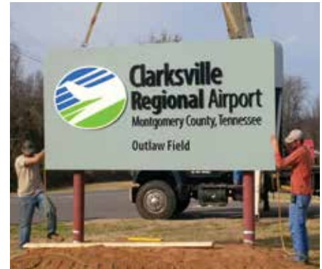
Installation – Main ID Sign
